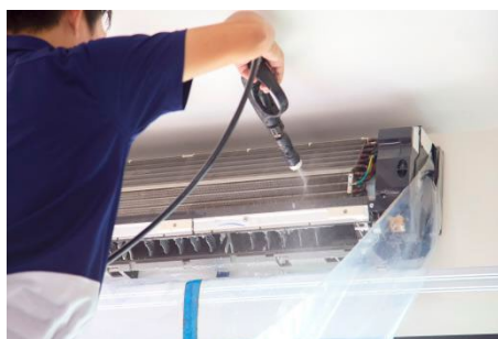
Regular servicing boosts AC performance
